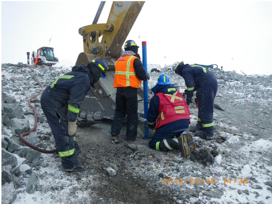
Photo 3: Inclinometer casing back-filling operations.
