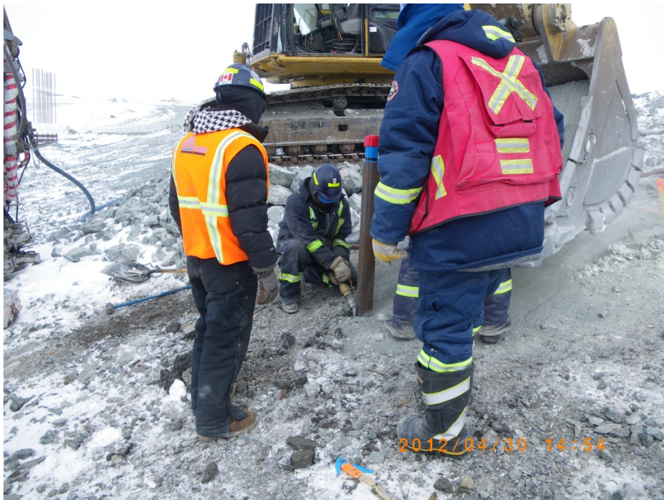
Photo 4: The 4" Sced 40 protective housing installed. The Inclinometer casing to be cut to final elevation and the protective steel cover yet to be manufactured.
